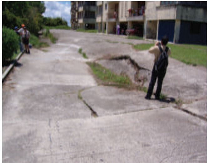
Damages captured in 2008 at the Kundasang High School attributed to the Mensaban and Loubo-Loubo active faults.
